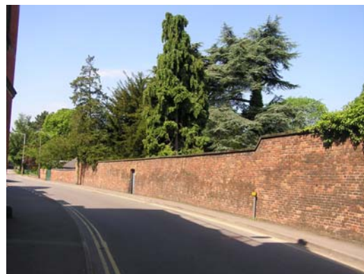
High brick boundary wall in Ashbourne
