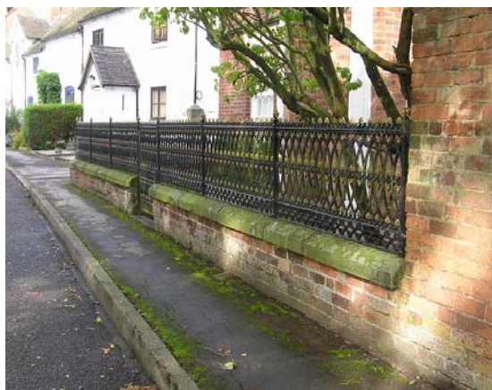
Decorative railings in Clifton
