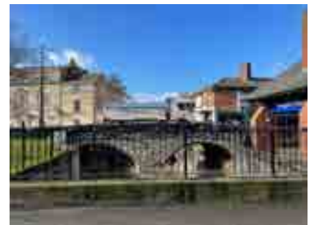
Figure 38: Dig Street Bridge
