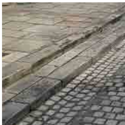
Figure 27: Yorkstone paving and kerbs
