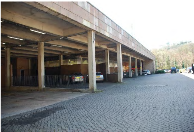
3. Former bus station – lean to roof structure
