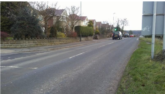
(Photograph 8 – View north east from Chesterfield Road at the Wolds Road Junction)
