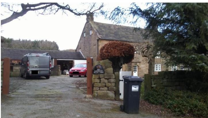
(Photograph 18 – The Wolds Farm House – Grade II Listed)
