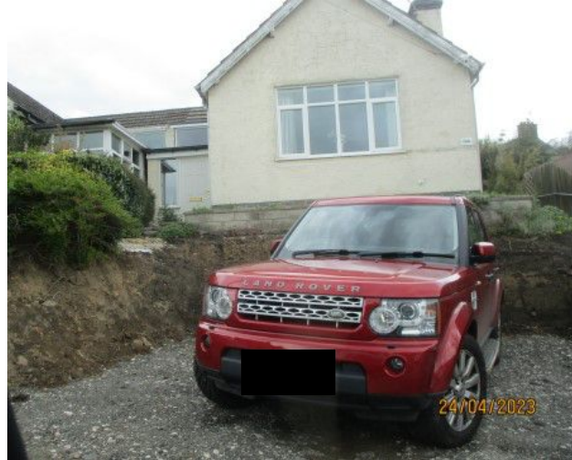
Site following works.
